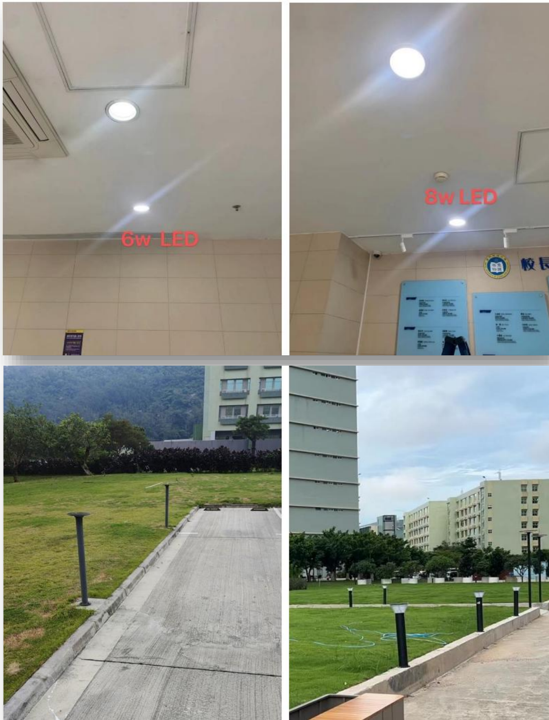
Fig. 11 LED energy-saving lights and outdoor PV lights on campus
